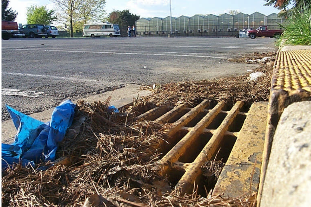
Figure 2-11 Impervious Surface is created with new urban growth. Impervious surface carries significant implications for water quality and flooding as non-point source pollution and runoff are greatly increased.
