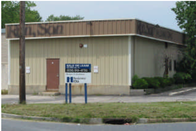
Figure – 25a The old mushroom factory is a building that could be redeveloped as part of a technology center.
