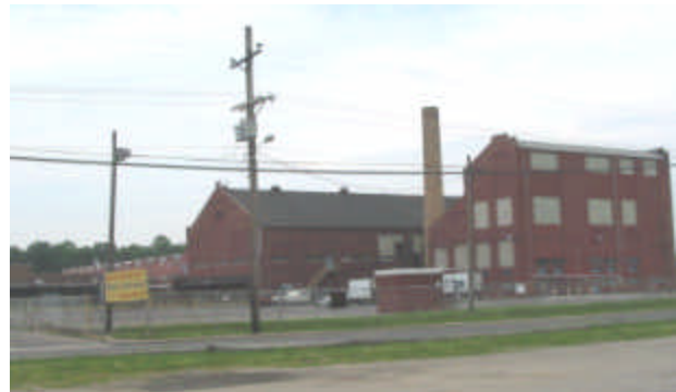
Figure – 25b – The old Glassboro glass factory would make an excellent redevelopment site for the south Jersey technology park. It is within close proximity to the main campus, the downtown redevelopment district and potential light rail on the existing Conrail tracks.
