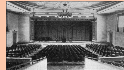
Historic Tobill Auditorium now holds student theater and dance productions, but the 2002 addition to Wilson Hall will provide for all Fine and Performing Arts performances under one roof.
