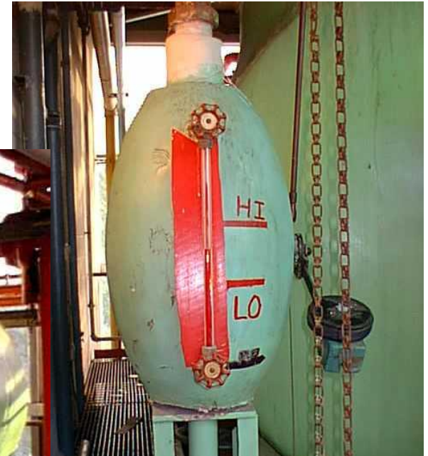
Liquid Level Indicator Remember \rho gh !
