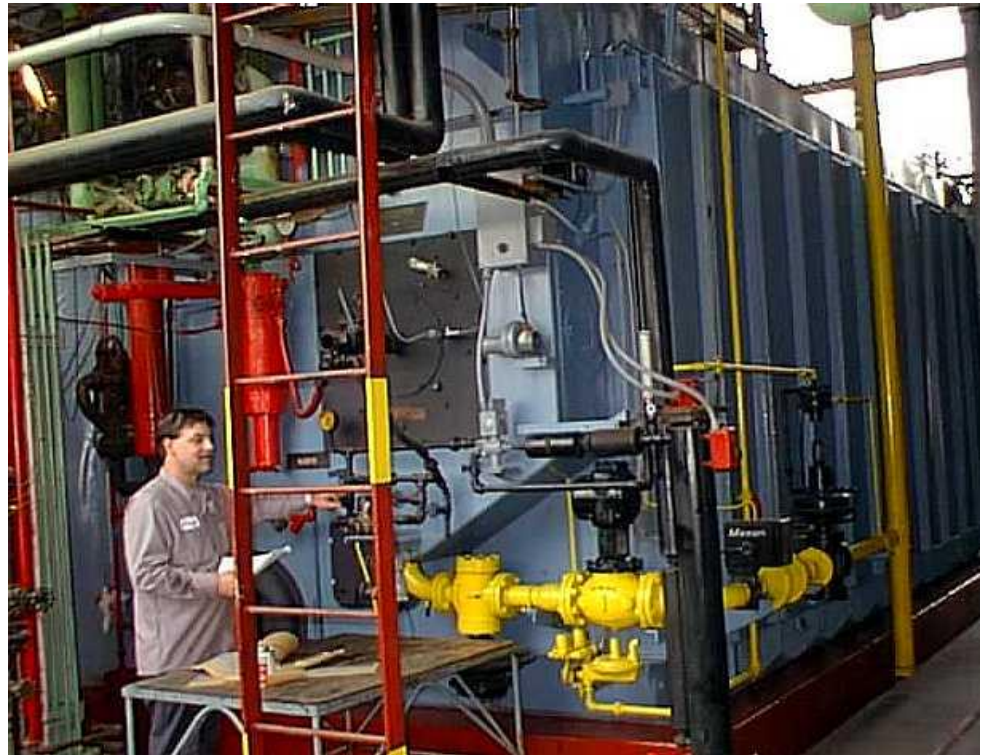
Conventional Boiler Unit
