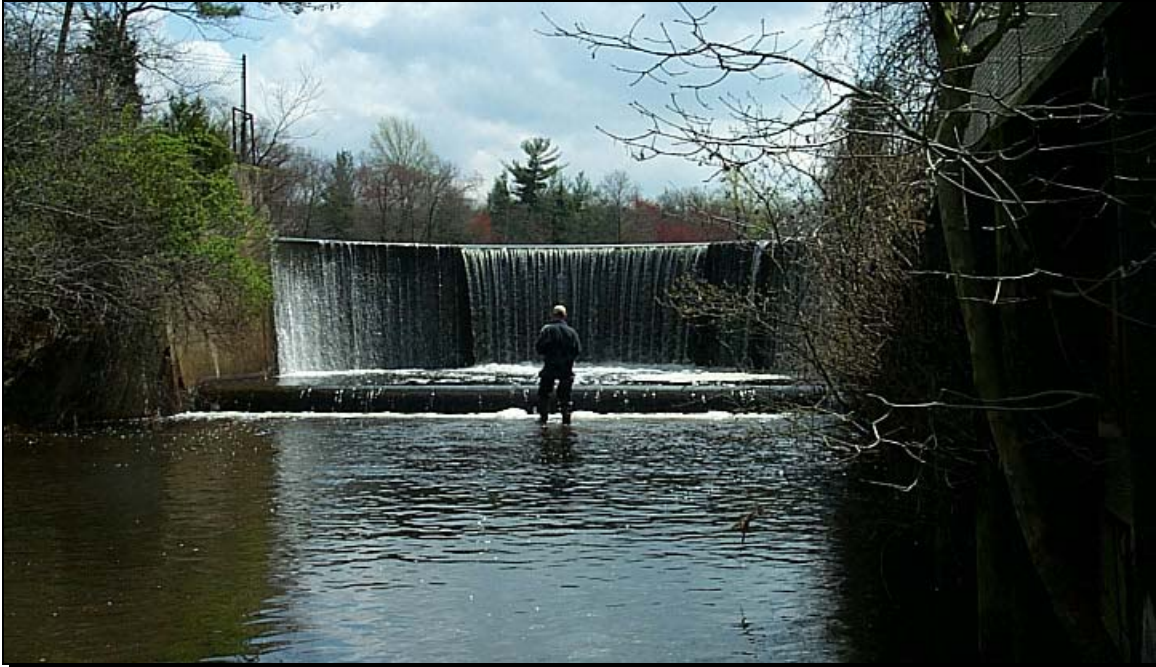
Figure 4: The spillway at Wadsworth Dam, looking upstream.
